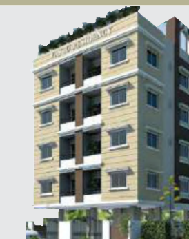
VASTU RESIDENCY - I Shahu Nagar, Manewada
